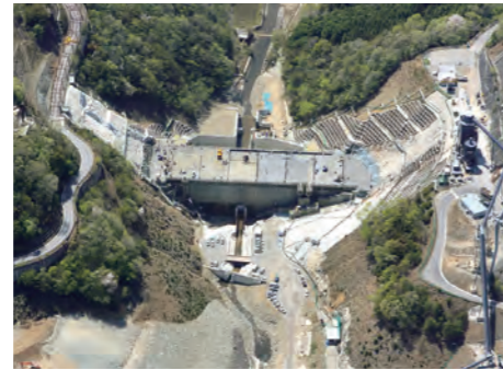
②⑥ 堤体打設状況(全面レア)(H26.4)
